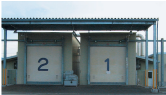
燻蒸施設 Fumigation Warehouse
