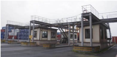
IN / OUT GATE
