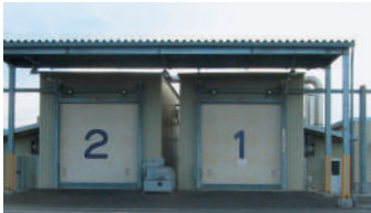
燻蒸施設 Fumigation Warehouse
