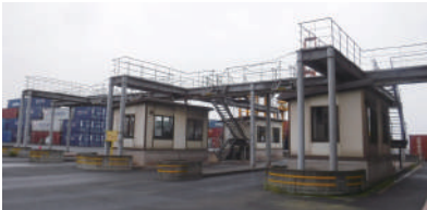
IN / OUT GATE
